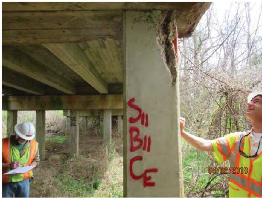
BENT 11 - AT COLUMN E
