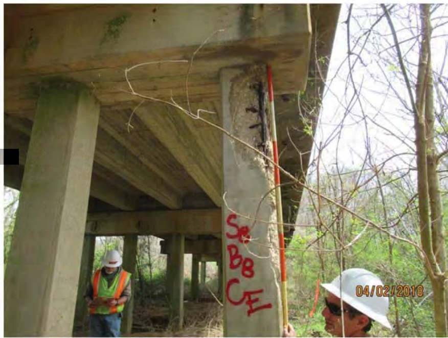
SPAN 8 - BENT 8 - COLUMN E
