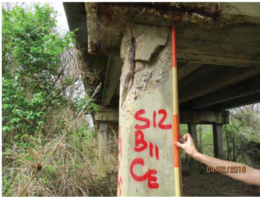
SPAN 12 - BENT 11 - COLUMN E
