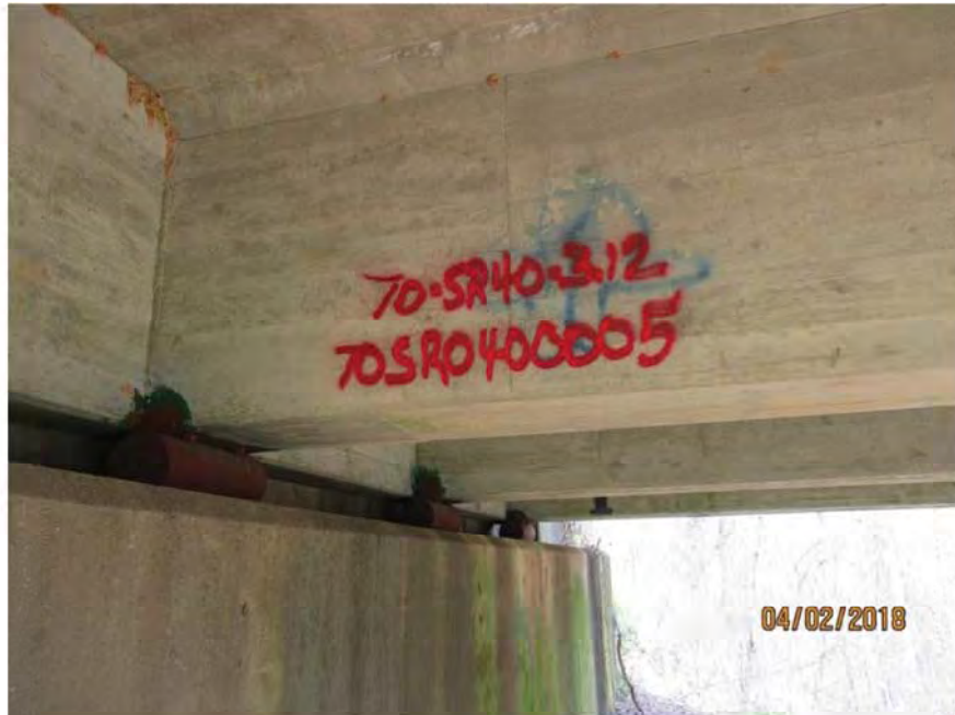
BRIDGE NUMBER - SPAN 1 - BEAM C
