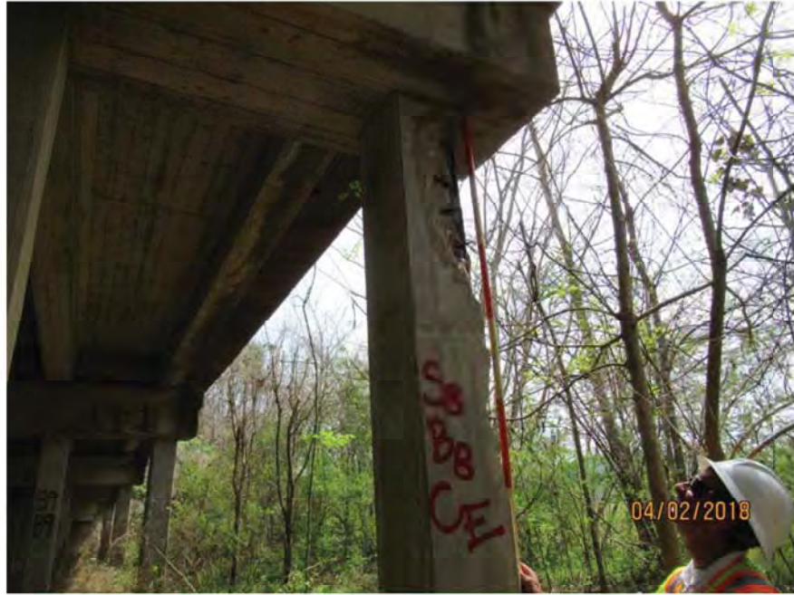
SPAN 8 - BENT 8 - COLUMN E
