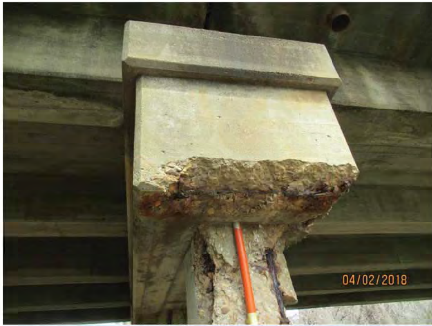
BENT 11 - AT COLUMN E - CAP
