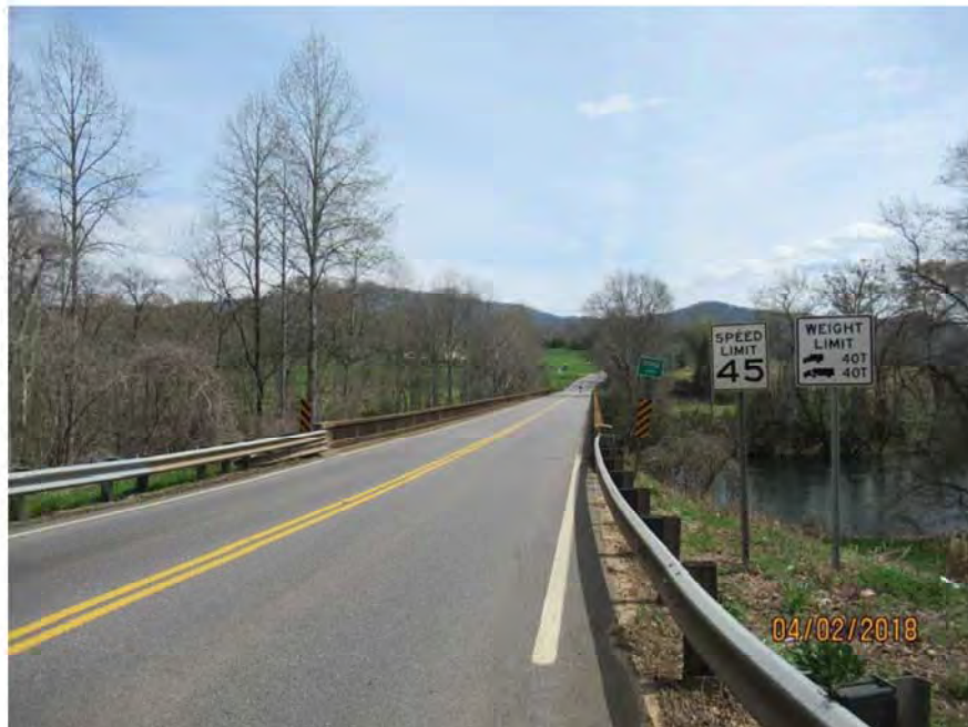
LOOKING AHEAD ON STRUCTURE - WEIGHT POSTING – TO NC
