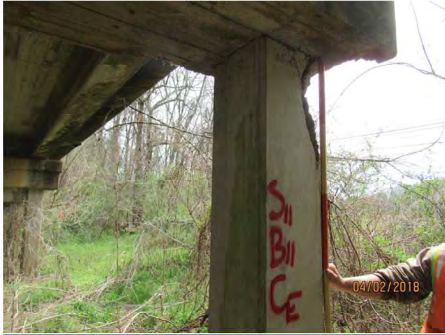
BENT 11 - AT COLUMN E
