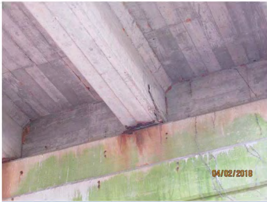
SPAN 7 - BENT 6 - BEAM B
