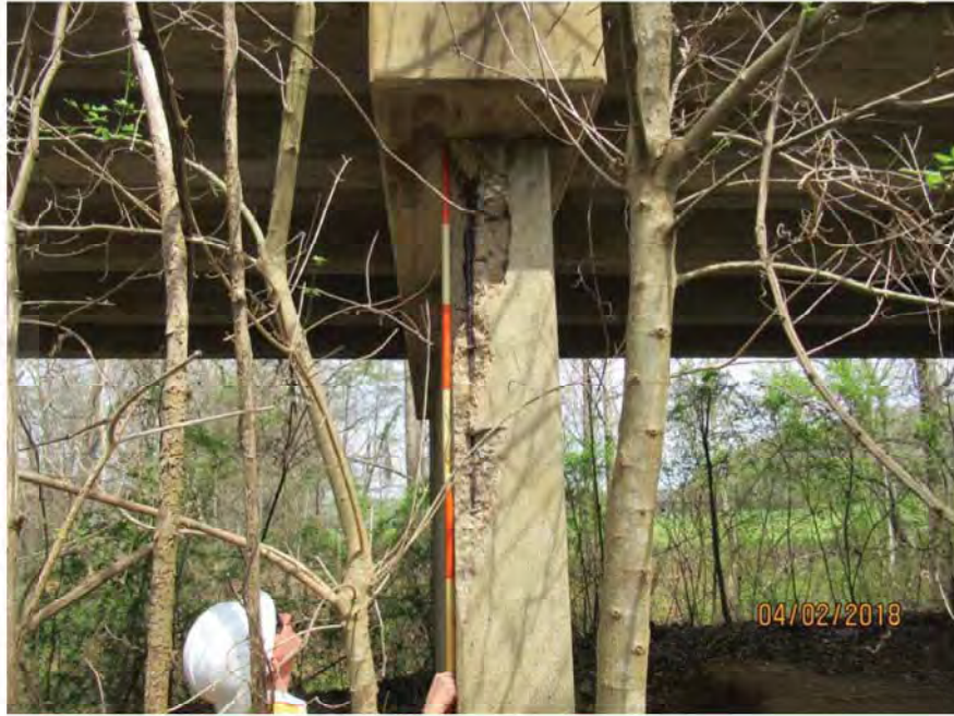
SPAN 8 - BENT 8 - COLUMN E
